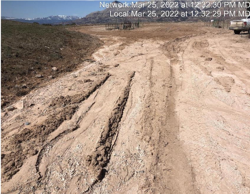
Photo #6297 Sediment has been transported on to location.
