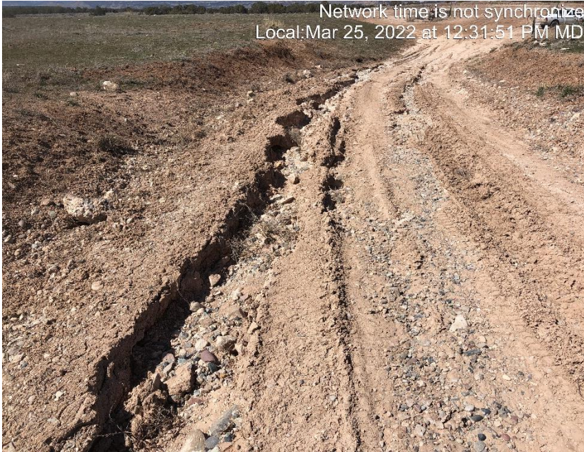
Photo #6294 Access road lacks stabilization.
