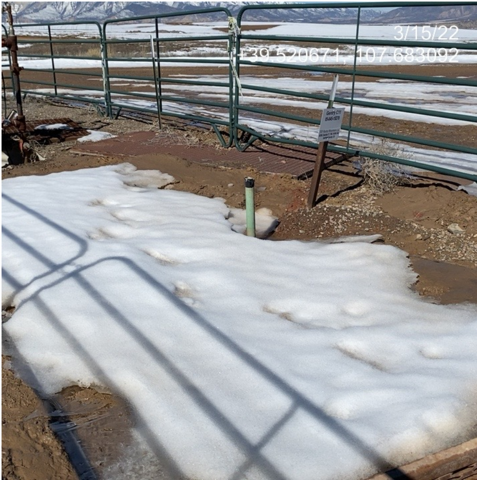
Photo 1. Photo shows reclaimed AL well API# 05-045-15270 with a pipe present.
