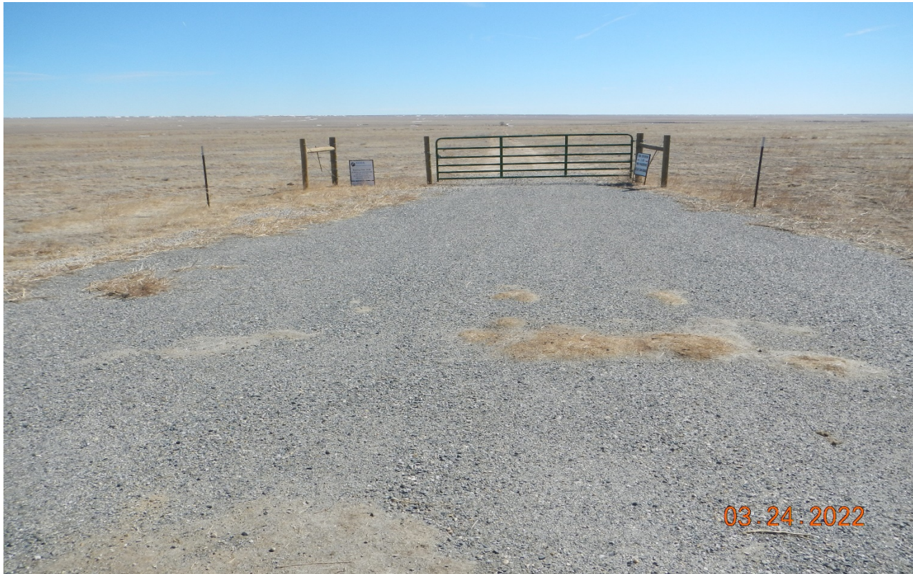
Photo 1. Facing east at the beginning of the access road. If well is plugged and abandoned the gravel will need to be removed and road will need to be reclaimed.
