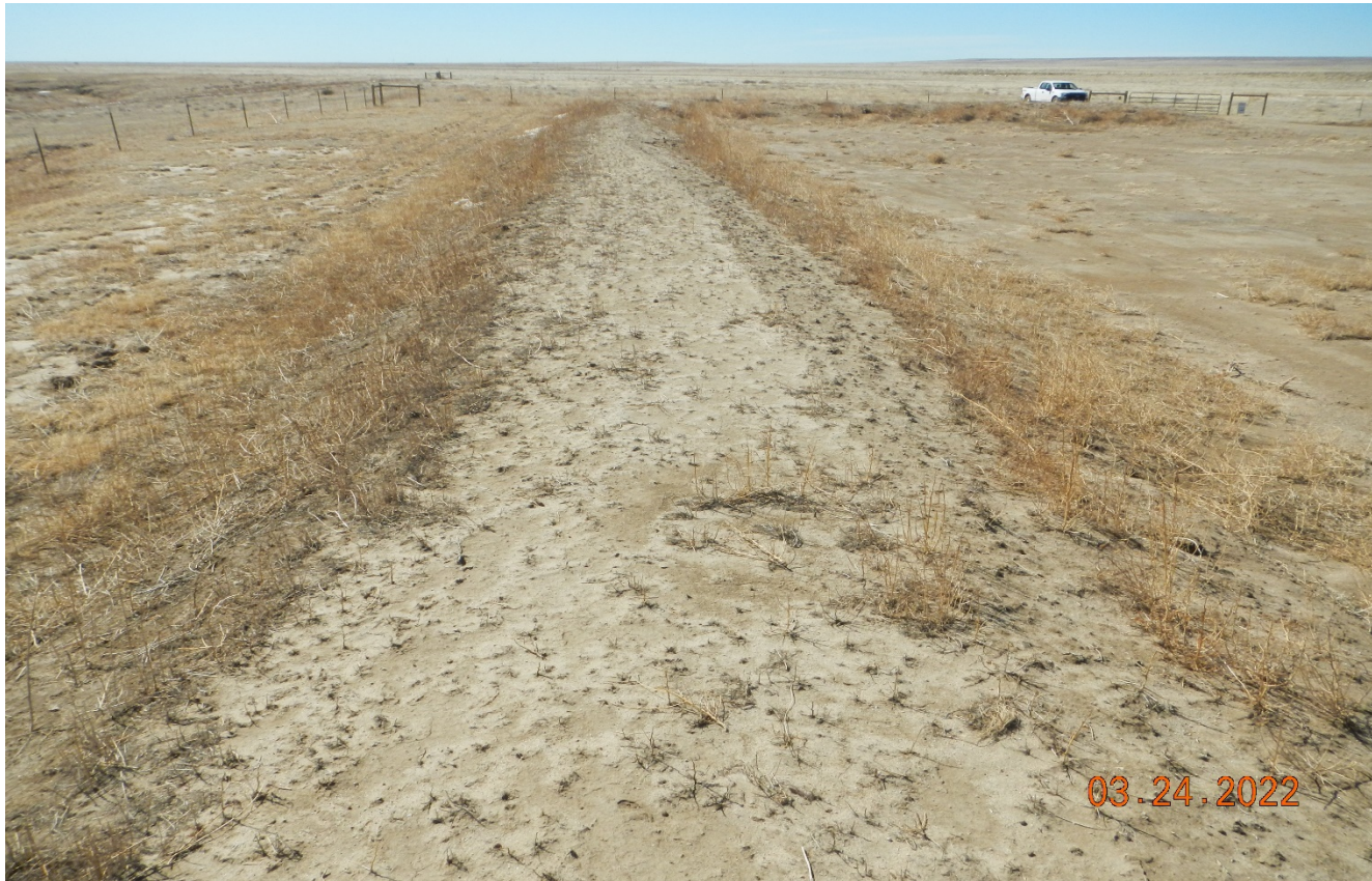
Photo 7. The topsoil pile stored along the perimeter are not protected from erosion and weed infestation. There are undesirable weeds throughout the topsoil piles.
