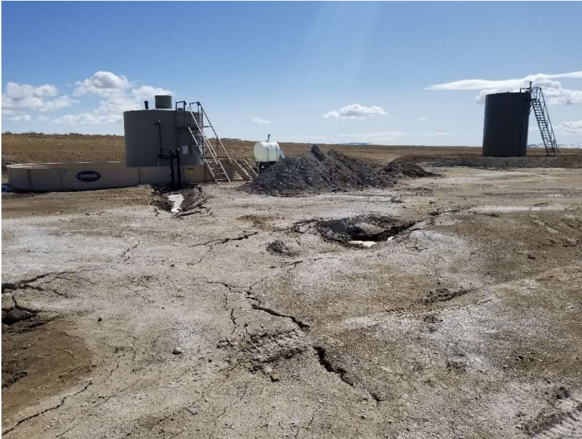
Photo 3. Subsidence on location. Soil piles without stormwater controls.
