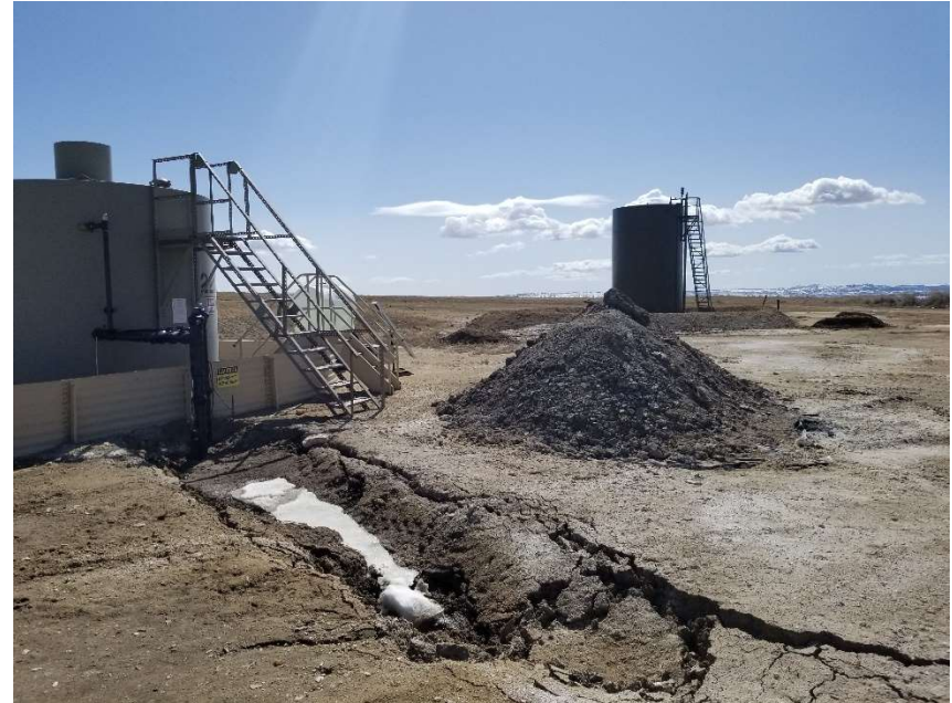
Photo 4. Subsidence on location. Soil pile without stormwater controls.
