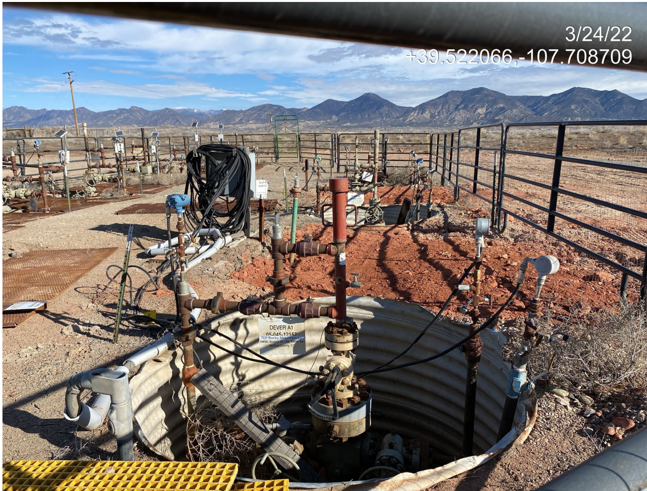
Photo 6. Photo taken from well area shows BMPs to prevent wildlife access to well cellars were missing or insufficient
