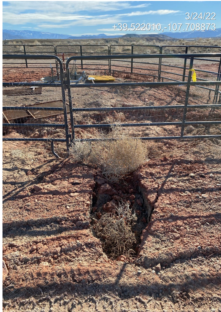
Photo 5. Photo taken from the wells facing east shows subsidence in a trench.
