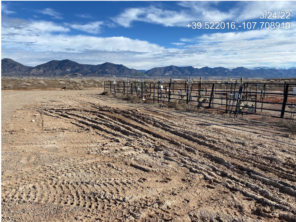
Photo 17. Photo taken from the west of the wells facing north shows rutting occurring on the pad.
