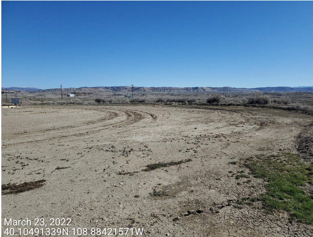
Photo 3: Photo example showing the production areas showing signs of destabilization; tracking/rutting becoming evident
