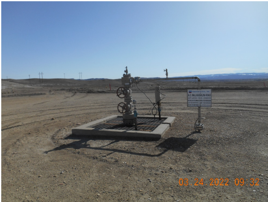
Injection wellhead
