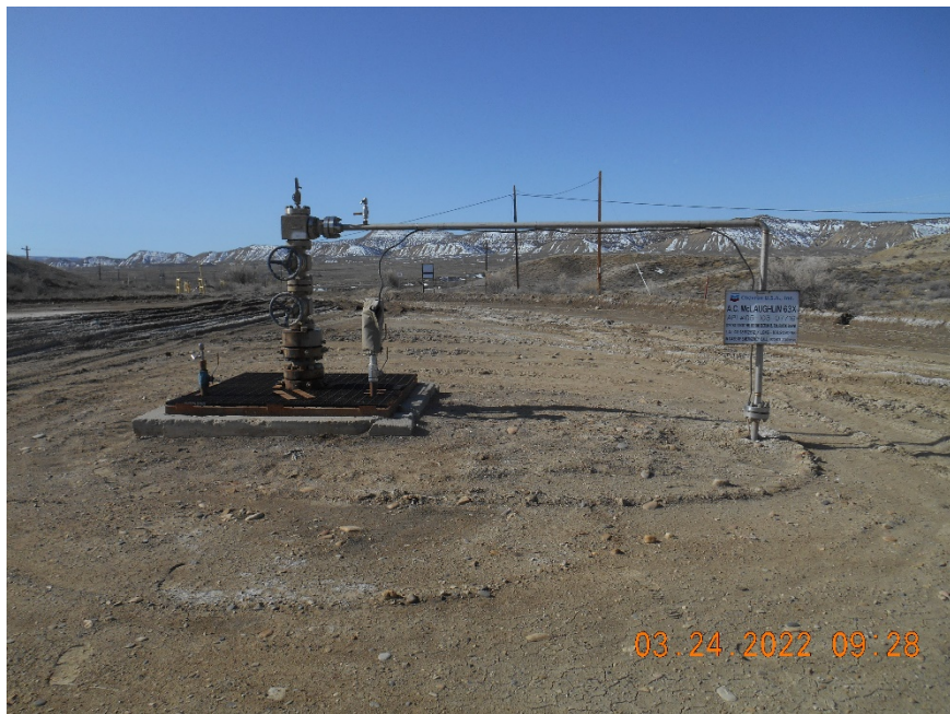
Injection wellhead
