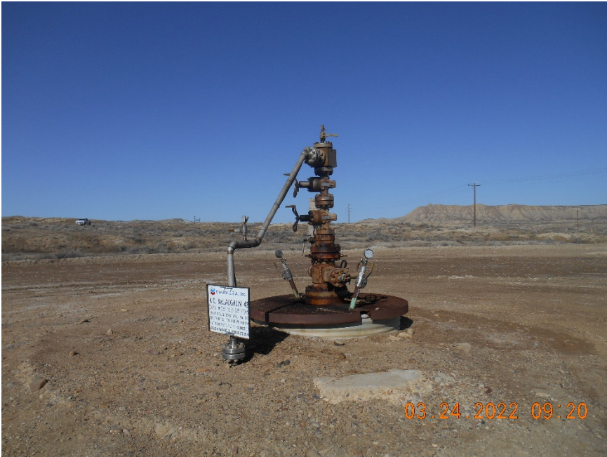
Injection wellhead
