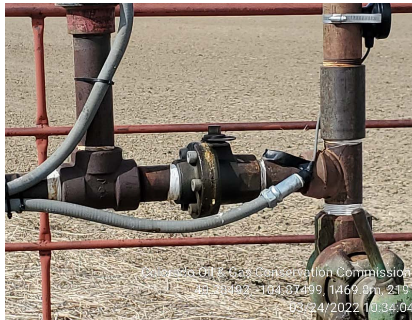
Valve leak
