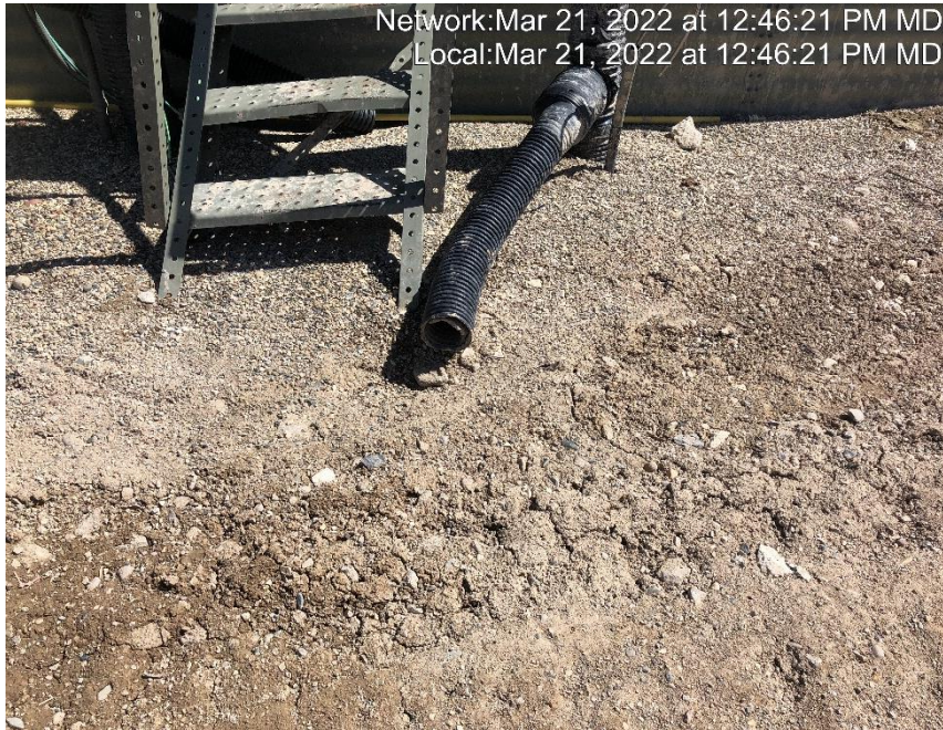
Photo #6257 flow line heating insulation open ended and not capped.
