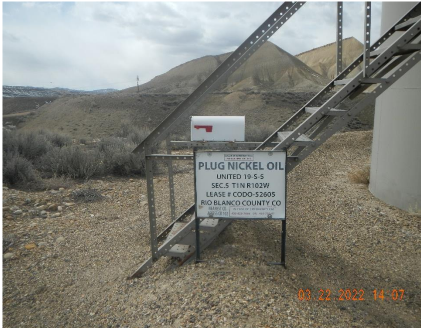
Tank battery sign has no API #
