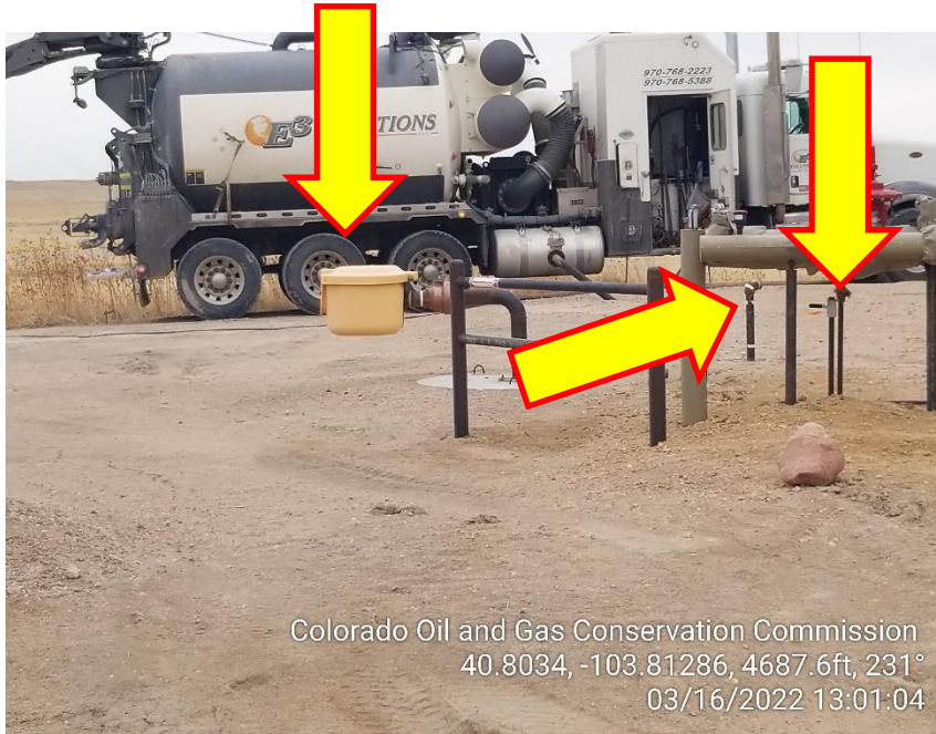
Photo 11 – Missing Labels – NFPA, Content and Capacity Unmarked Risers
