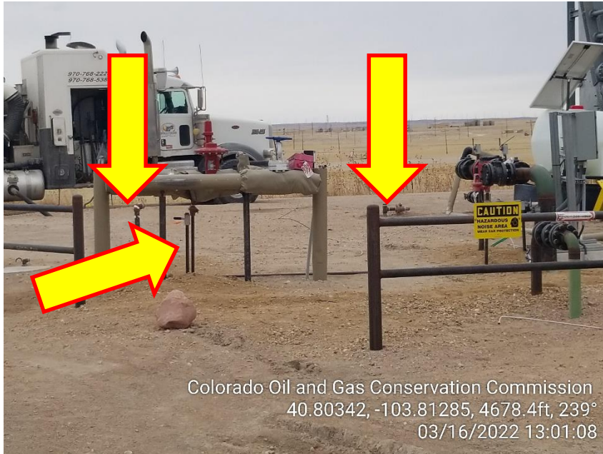
Photo 13 – Unmarked Risers
