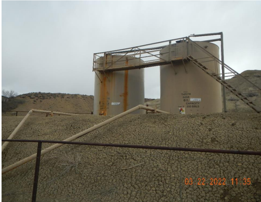
Damaged tank labels.
