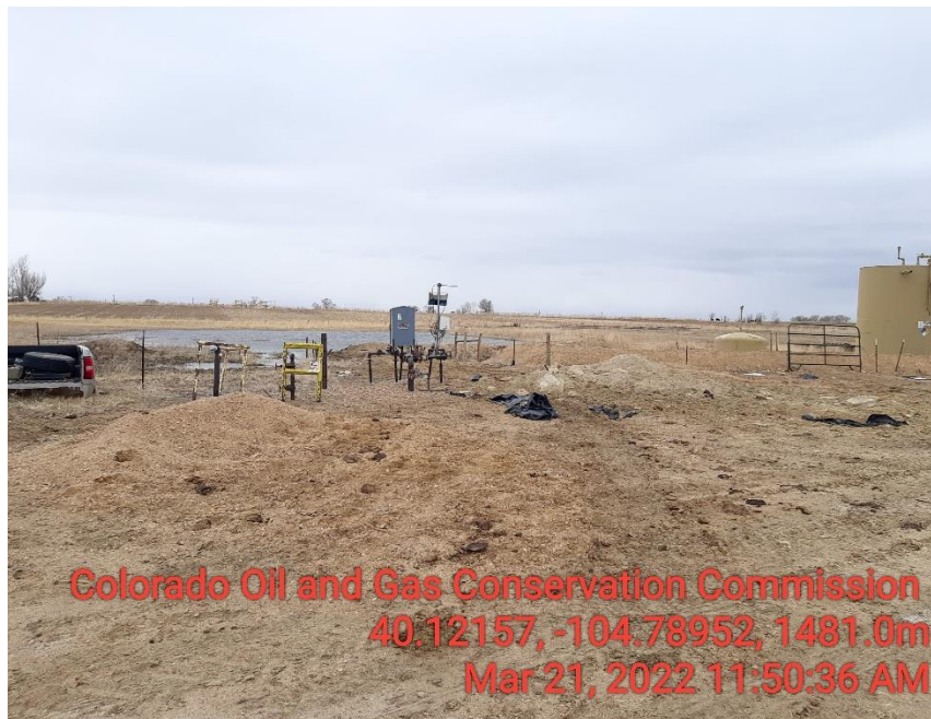
Photo 3 not BMP's or fencing around contaminated material
