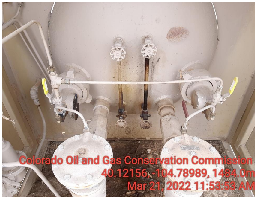
Photo 11 mechanical issue (sight Glass) and stained soil.
