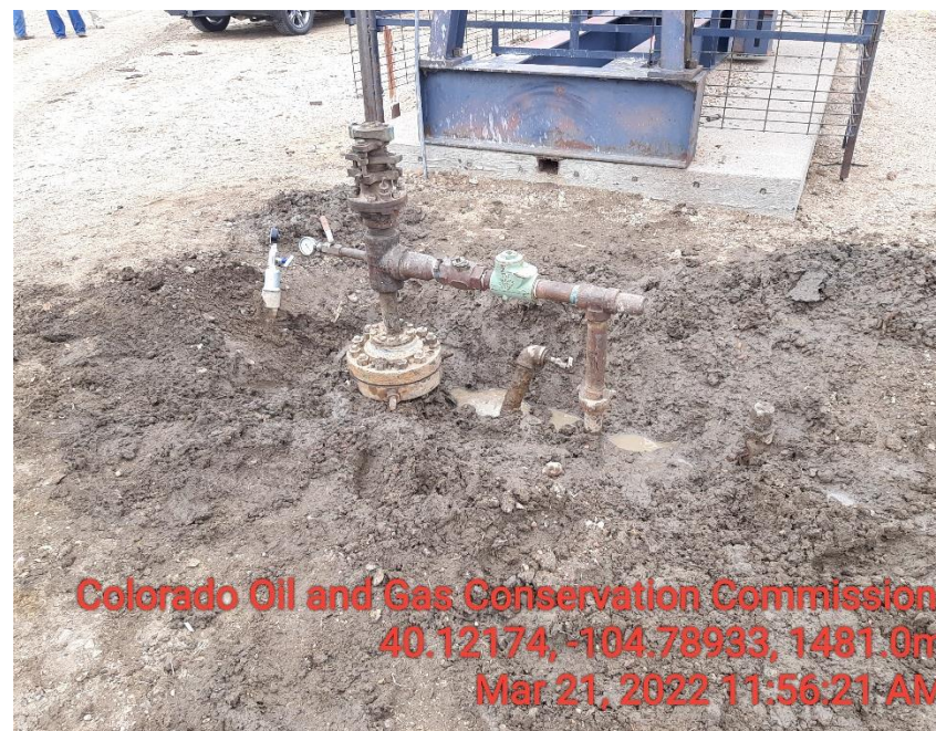
Photo 16 braden head test no gauge on braden head line.
