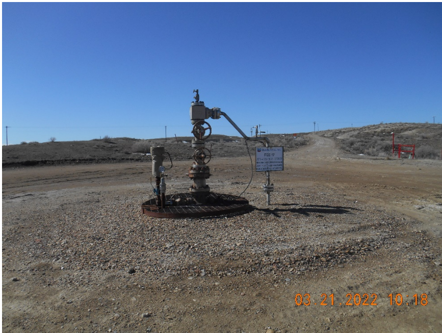
Injection wellhead
