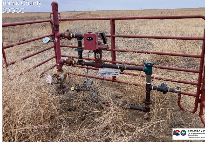
Pic 1 wellhead, at time of inspection one casing valve was slightly open and was put in the close position. Master valve is seized in position, unable to determine if valve was in open or close position. Ball valves on flowline are in close position.
