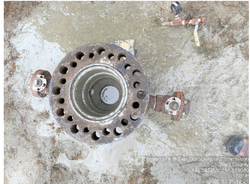
Photo #2 Dyer 2-21 Wellsite Plugged & Abandoned | PA Plugging Operations Cement to surface
