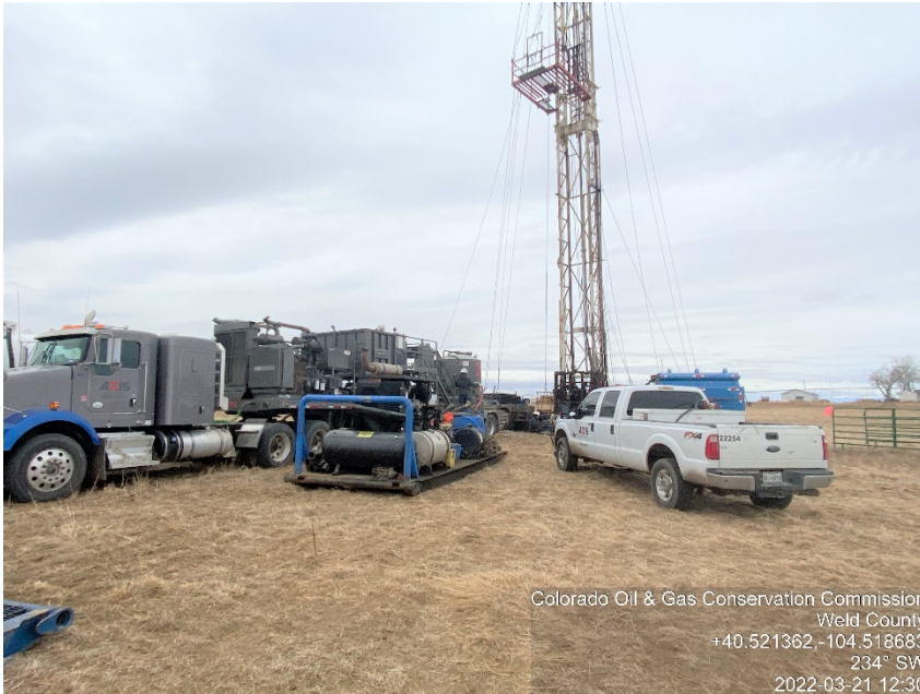
Photo #1 Dyer 2-21 (05-123-28012) Wellsite Plugged & Abandoned | PA Plugging Operations Cement to surface
