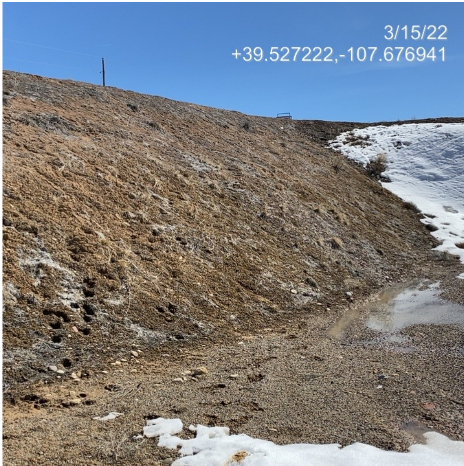
Photo 8. Photo taken from the east of the Location facing south shows unstabilized cut slopes.
