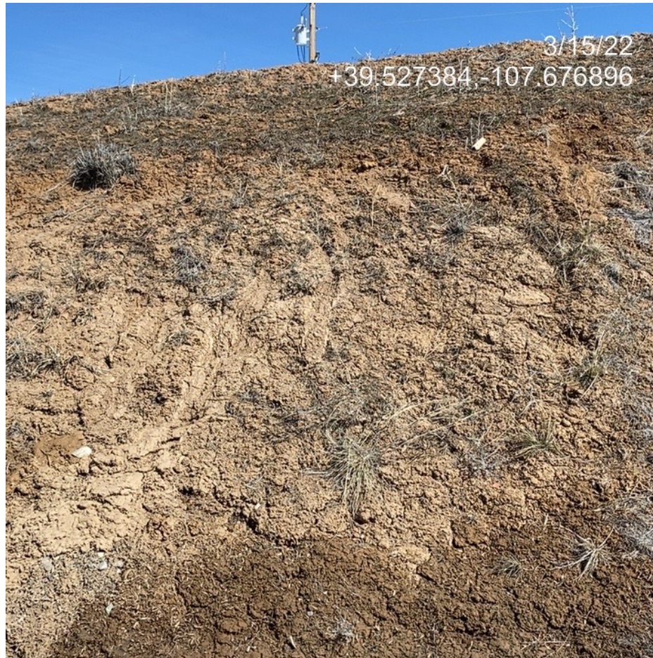
Photo 10. Photo taken from east of the Location shows rill erosion occurring on the unstabilized cut slope.
