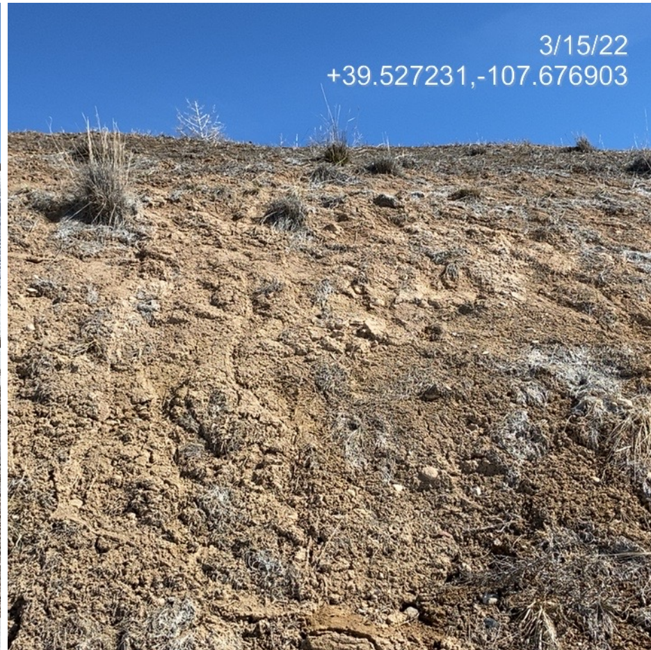
Photo 9. Photo taken from the east of the Location shows rill erosion occurring on the unstabilized cut slope.
