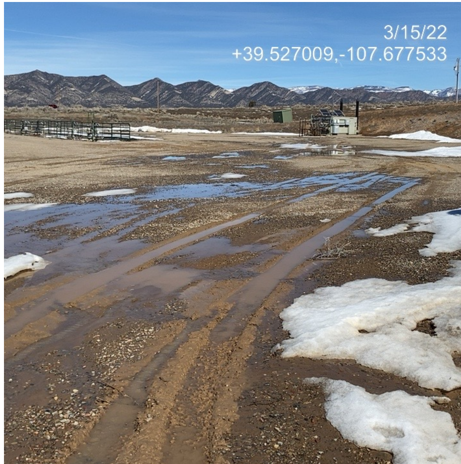
Photo 7. Photo taken from the entrance of the Location facing northeast shows rutting occurring on the pad.
