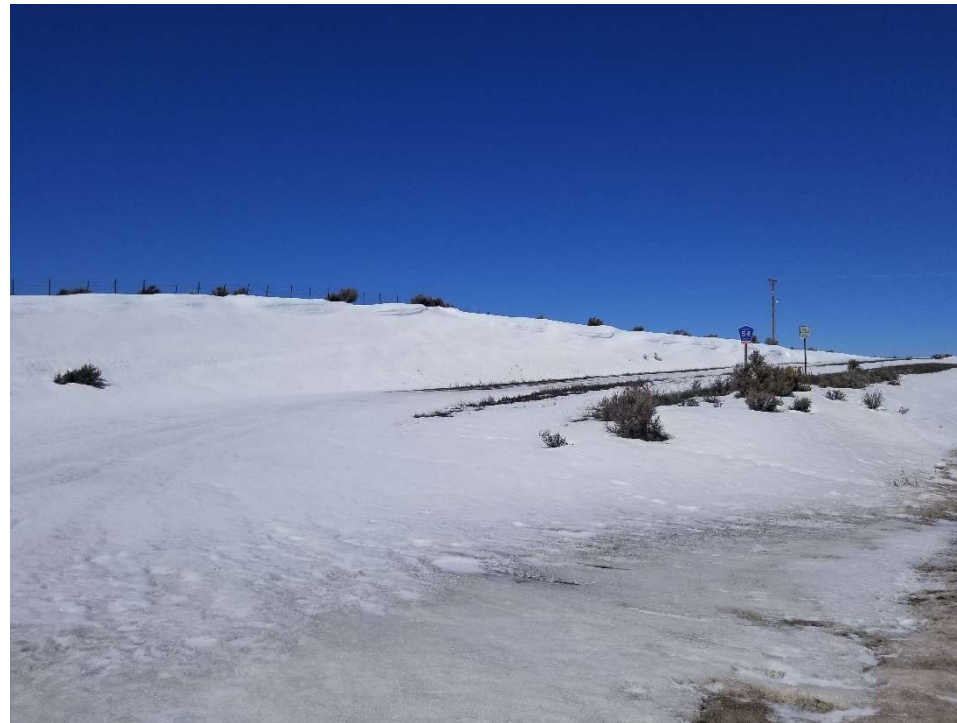
Photo 1. Roads not maintained for winter.
