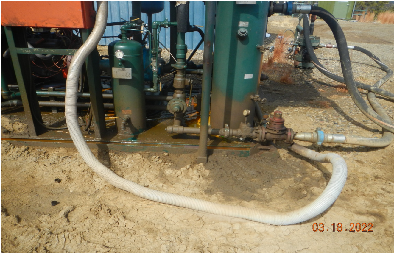
Photo 2. There is oily fluids in the engine skid and spill onto the ground.
