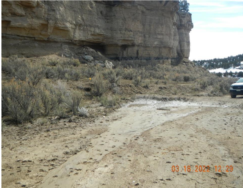
Sediment and storm water collecting at dirt berm across roadway..
