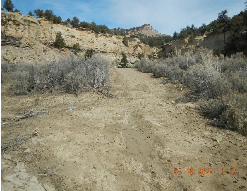
Washing on entrance road.
