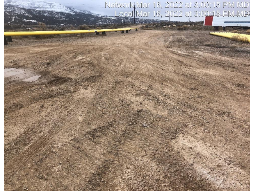
Photo #6225 Insufficient tracking controls at entrance to location.
