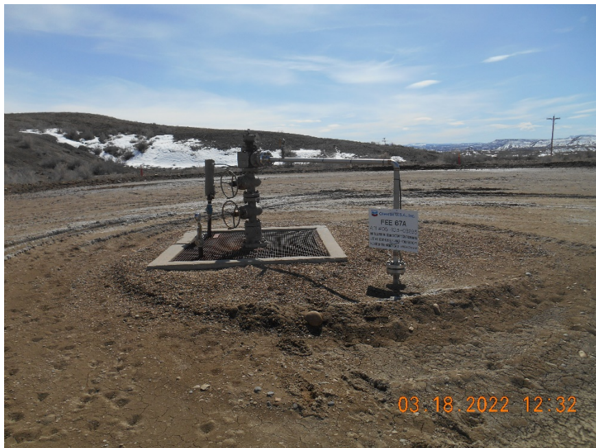
Injection wellhead
