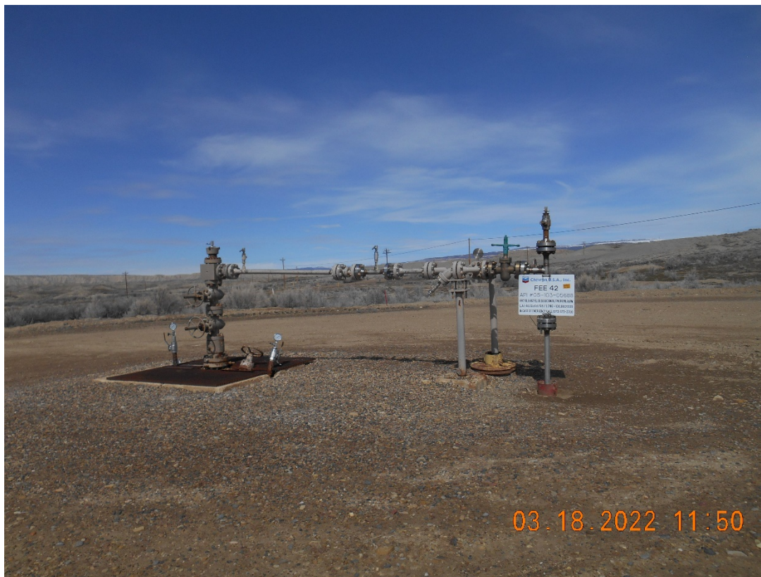
Injection wellhead- Temporarily Abandoned
