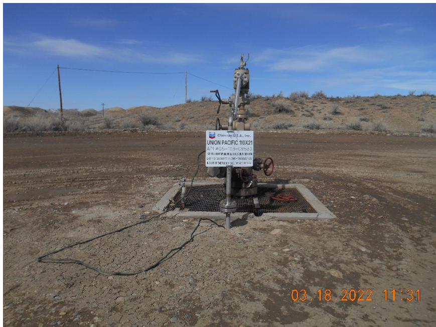
Injection wellhead
