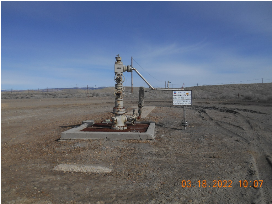
Injection wellhead
