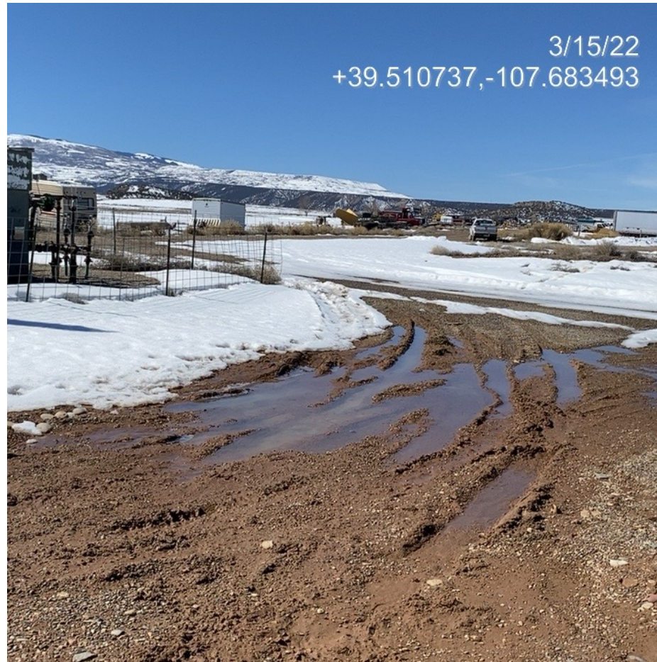
Photo 2. Photo taken from the southeastern production area facing west shows rutting occurring on the pad.
