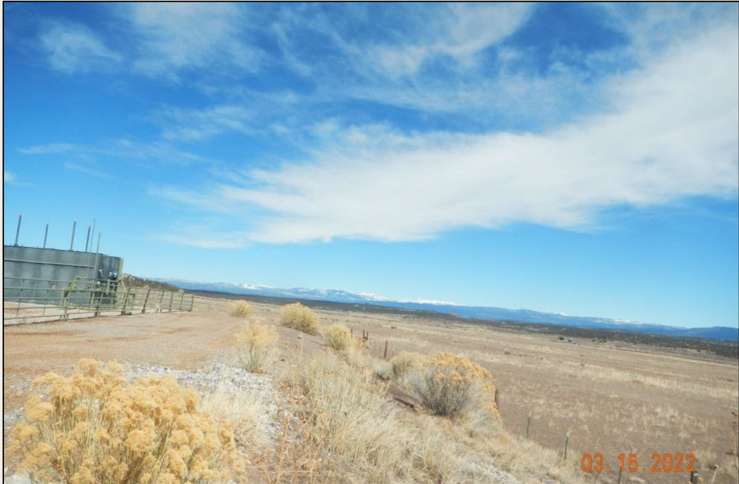
Photo 3. View of the eastern fill slope from the southeastern corner facing northward.
