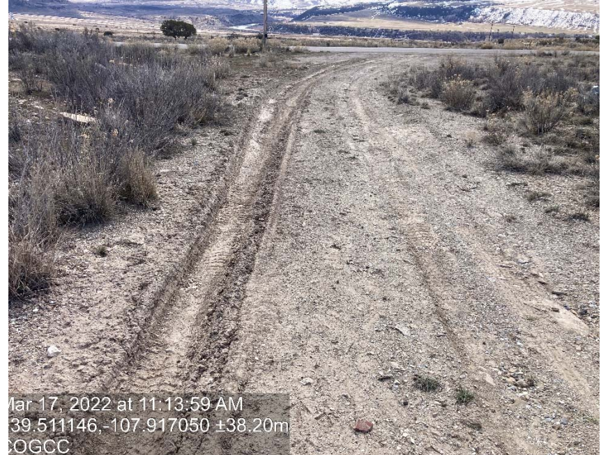
lack of stabilization/ compaction/ degrading.
