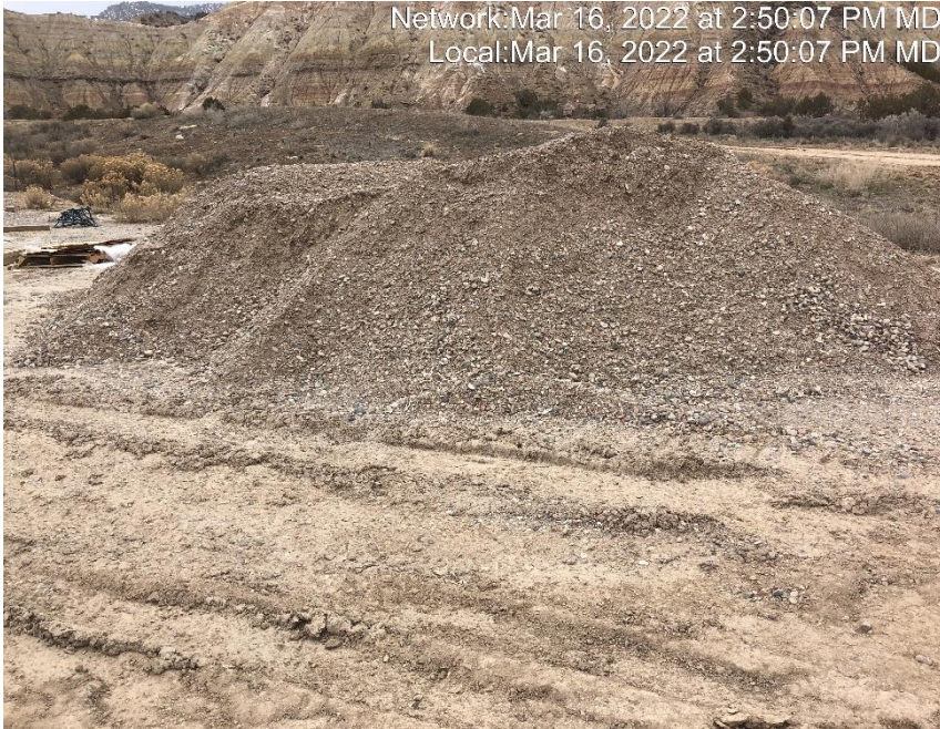
Photo #6216 Insufficient materials covering and BMP implementation.
