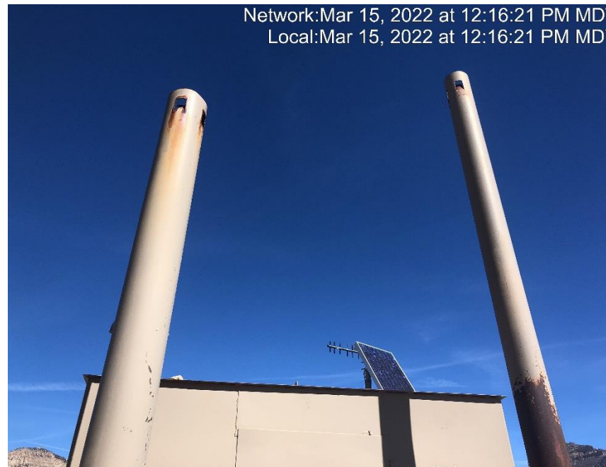
Photo #6171 Bird protectors missing on separator burners.
