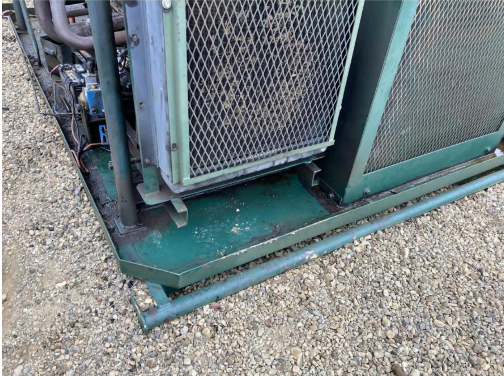
PHOTO 2: THE OILY FLUID ACCUMULATION AND RAGS HAVE BEEN REMOVED FROM THE CONTAINMENT. THE SELF INSPECTION PROCESS HAS BEEN REVIEWED
