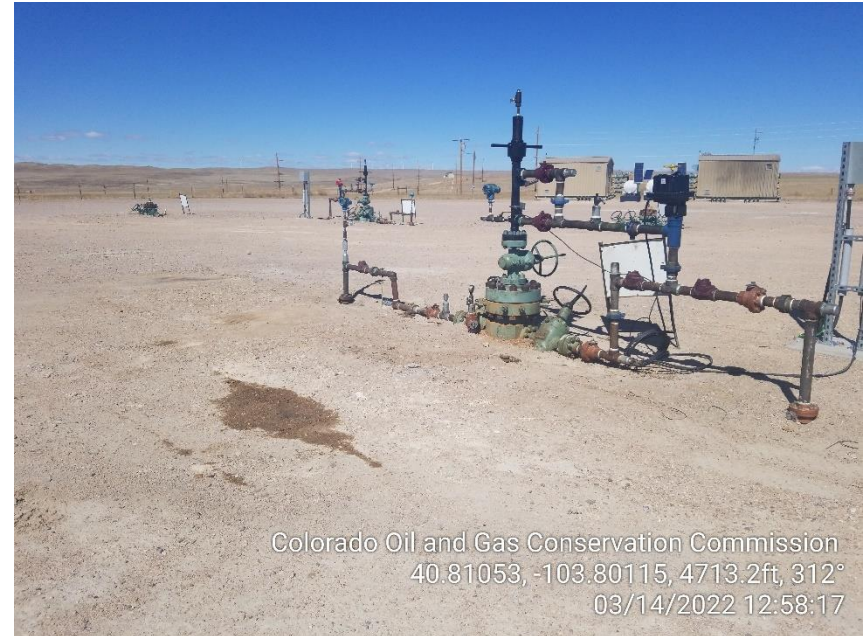
Photo 2 – Stained Soil at 3135 Wellhead
