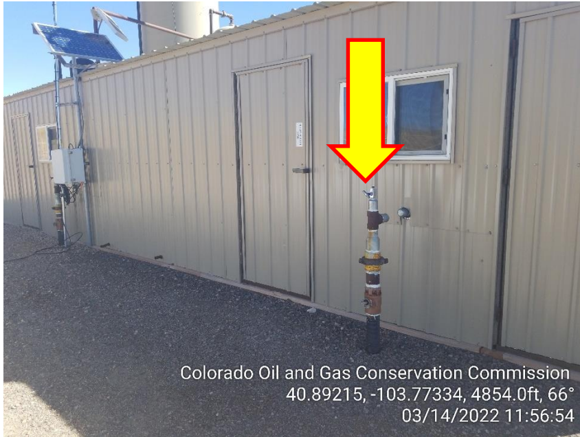
Photo 3 – Unmarked Riser
