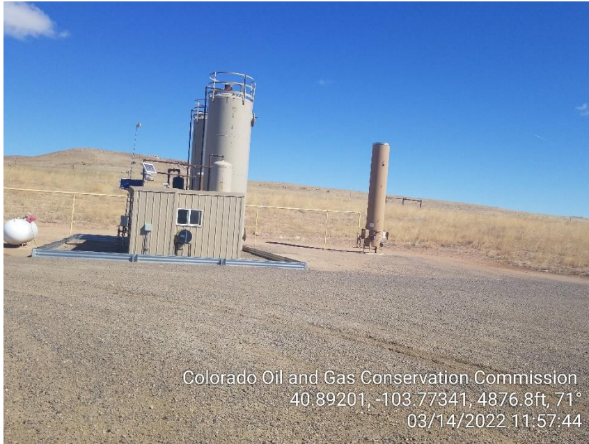
Photo 5 – Heater Treaters and ECD
