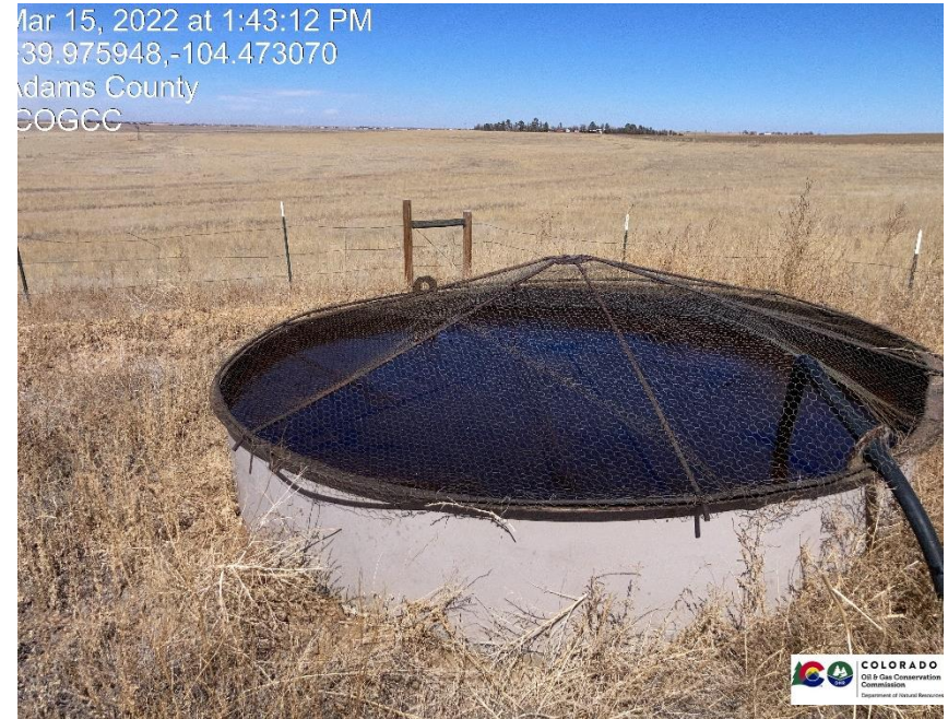
Pic 4 open top tank has fluid about 6" from top of tank, fluid needs to be removed before precipitation causes a spill
