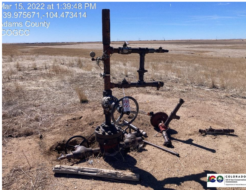
Pic 1 wellhead, at time of inspection all valves were in the close position. No bradenhead plumbed to surface, 2 missing bolts on wellhead,
