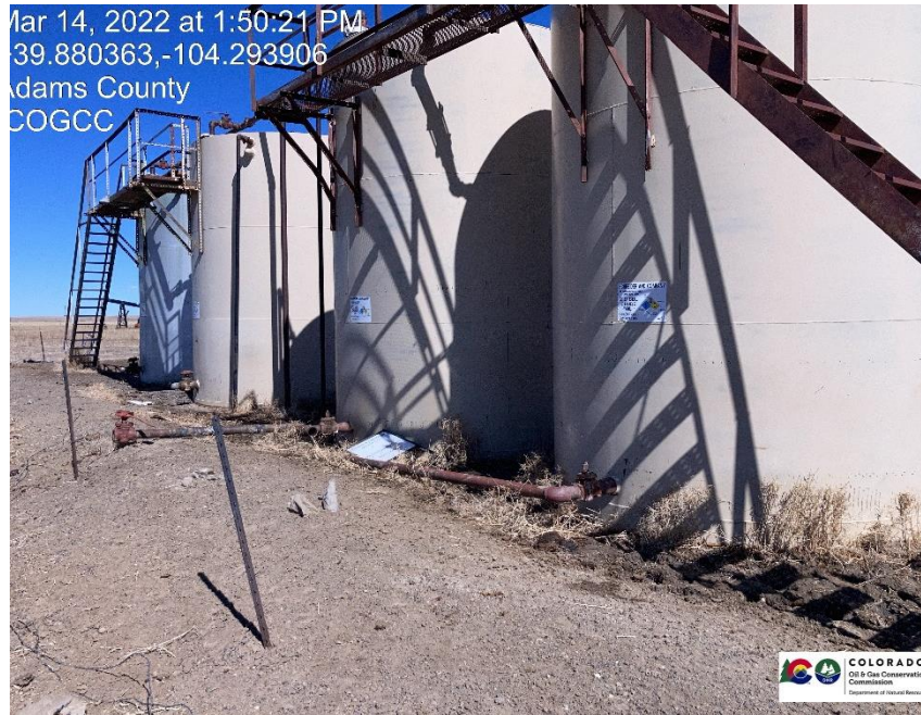
Pic 5 tanks, berms are not adequate.
