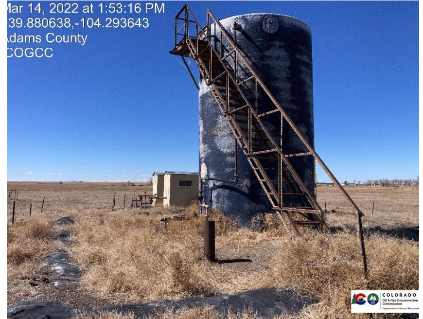
Pic 10 tank does not have any signage. Berms are not adequate.
