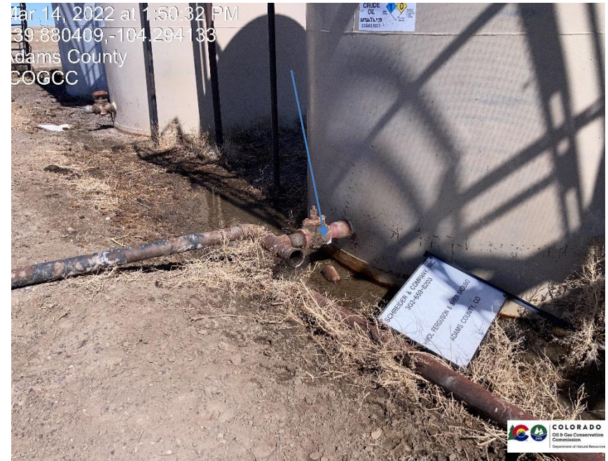
Pic 6 middle tank has a leak on valve
