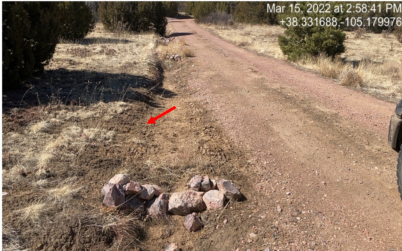
Photo 1. Facing northwest along the access road. The check dams along the road have filled in with sediment and need to be maintained.
