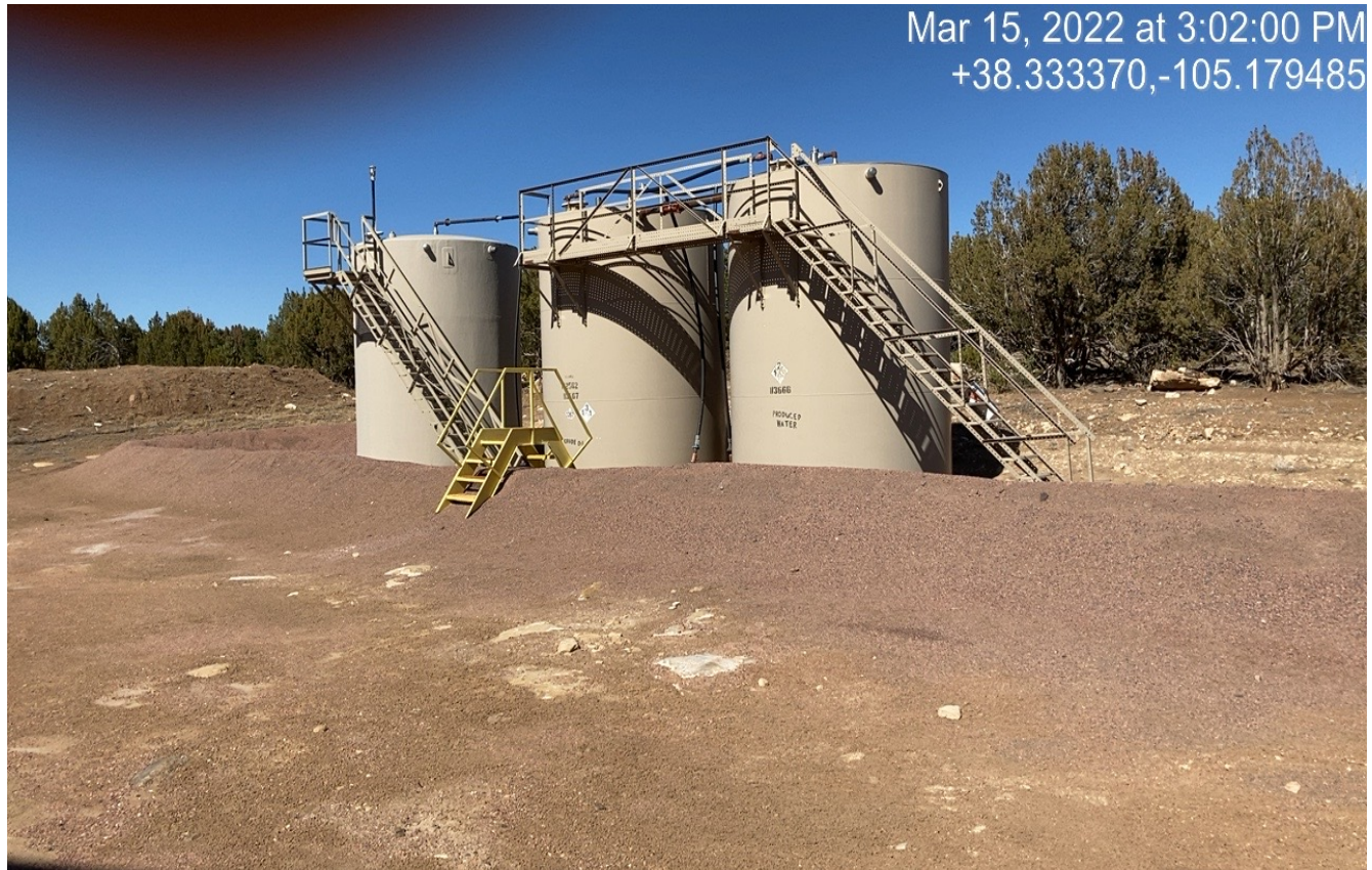
Photo 8. The tanks at north side of the location are not properly labeled.
