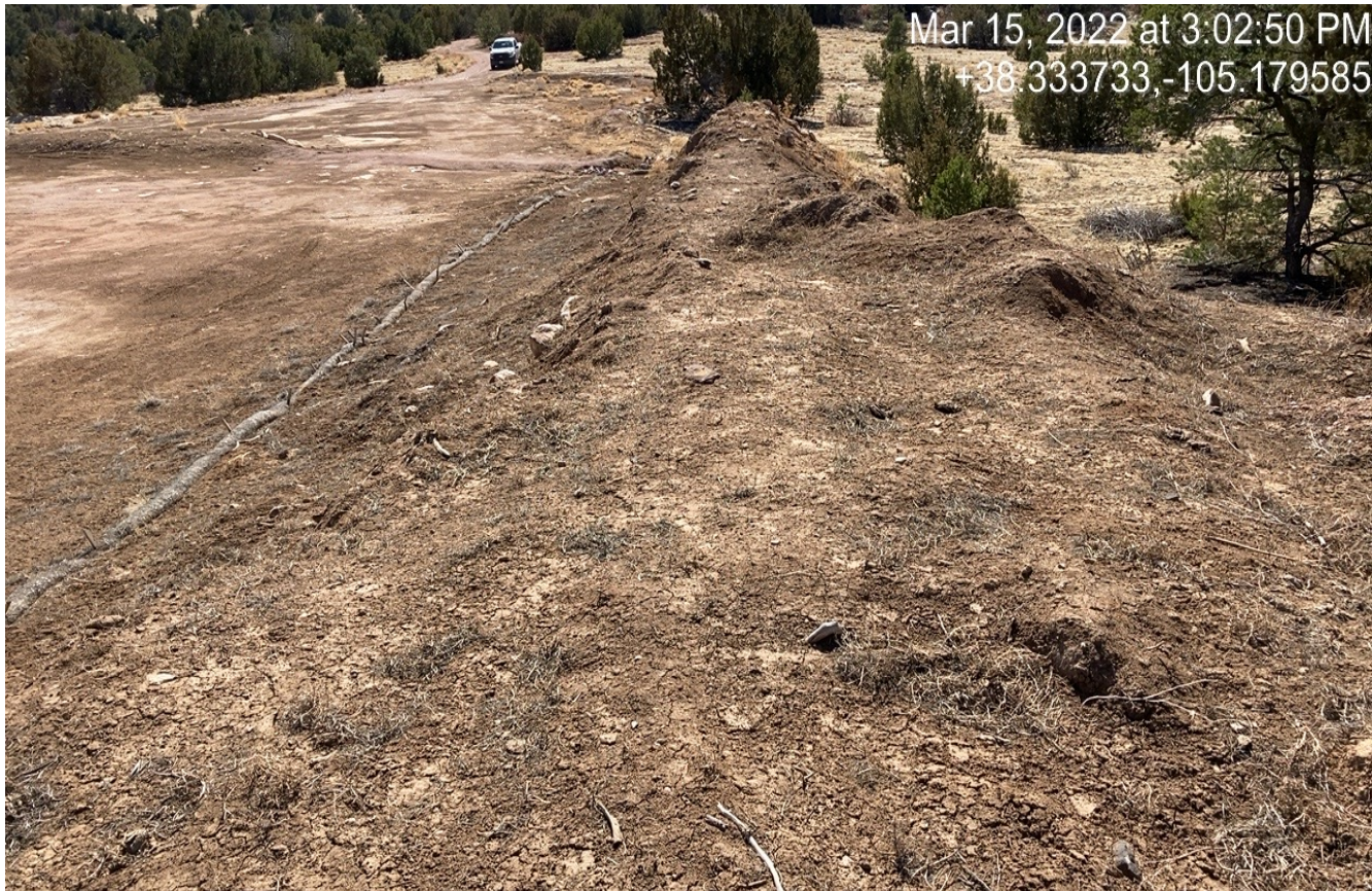
Photo 10. Facing toward the topsoil pile. The topsoil piles are not stabilized and protected. Topsoil piles have not been replaced for interim reclamation. Previous corrective action has not been performed.
