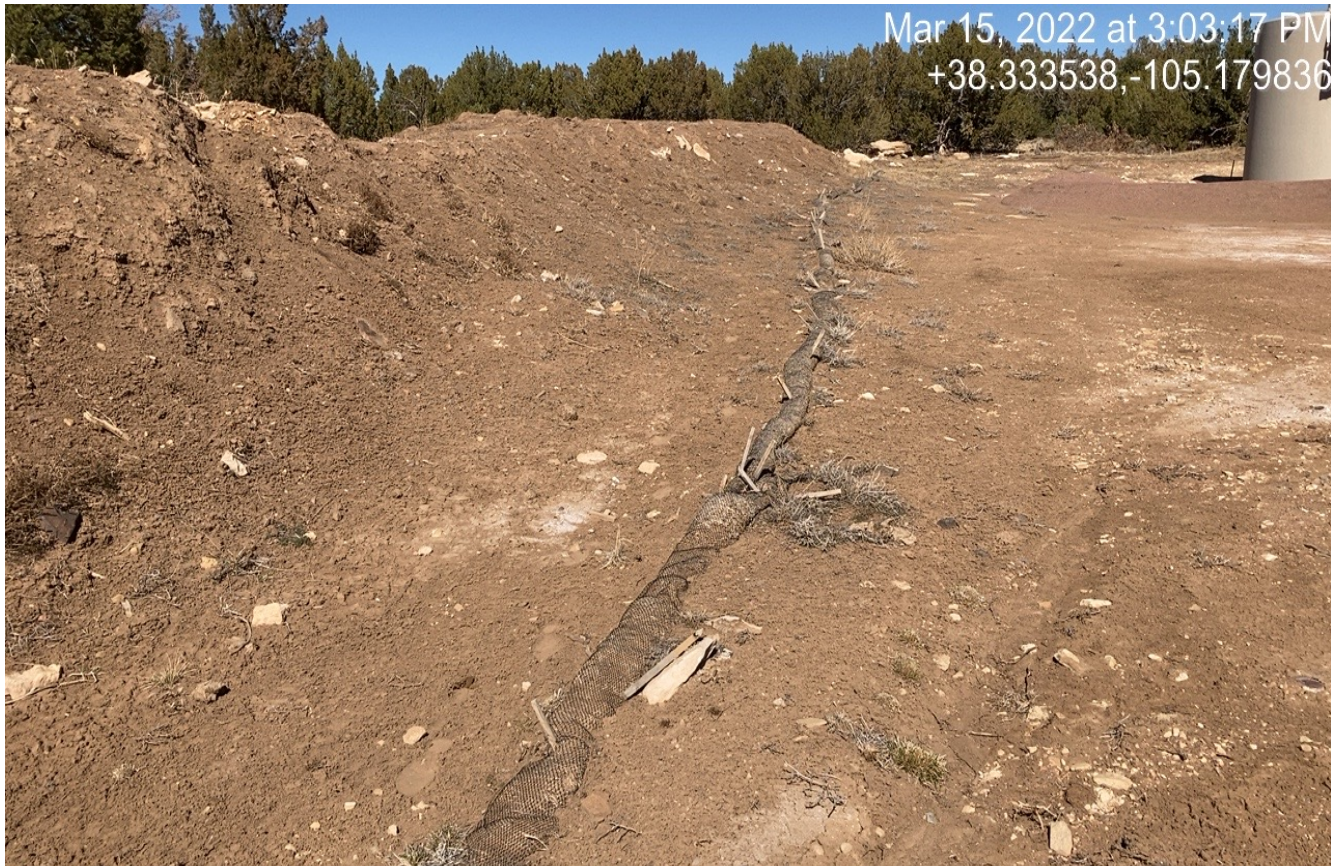
Photo 11. The wattles around the topsoil are degraded and not maintained.
