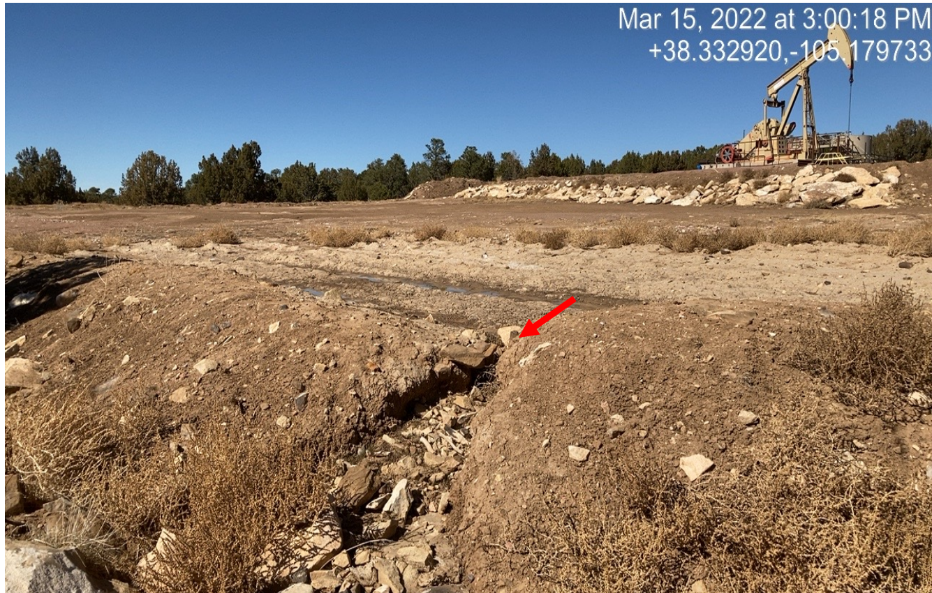
Photo 4. Facing northwest at the southeast corner of the location. There is erosion occurring from the disturbed pad site which is filling in the perimeter wattles. Previous corrective action has not been performed.
