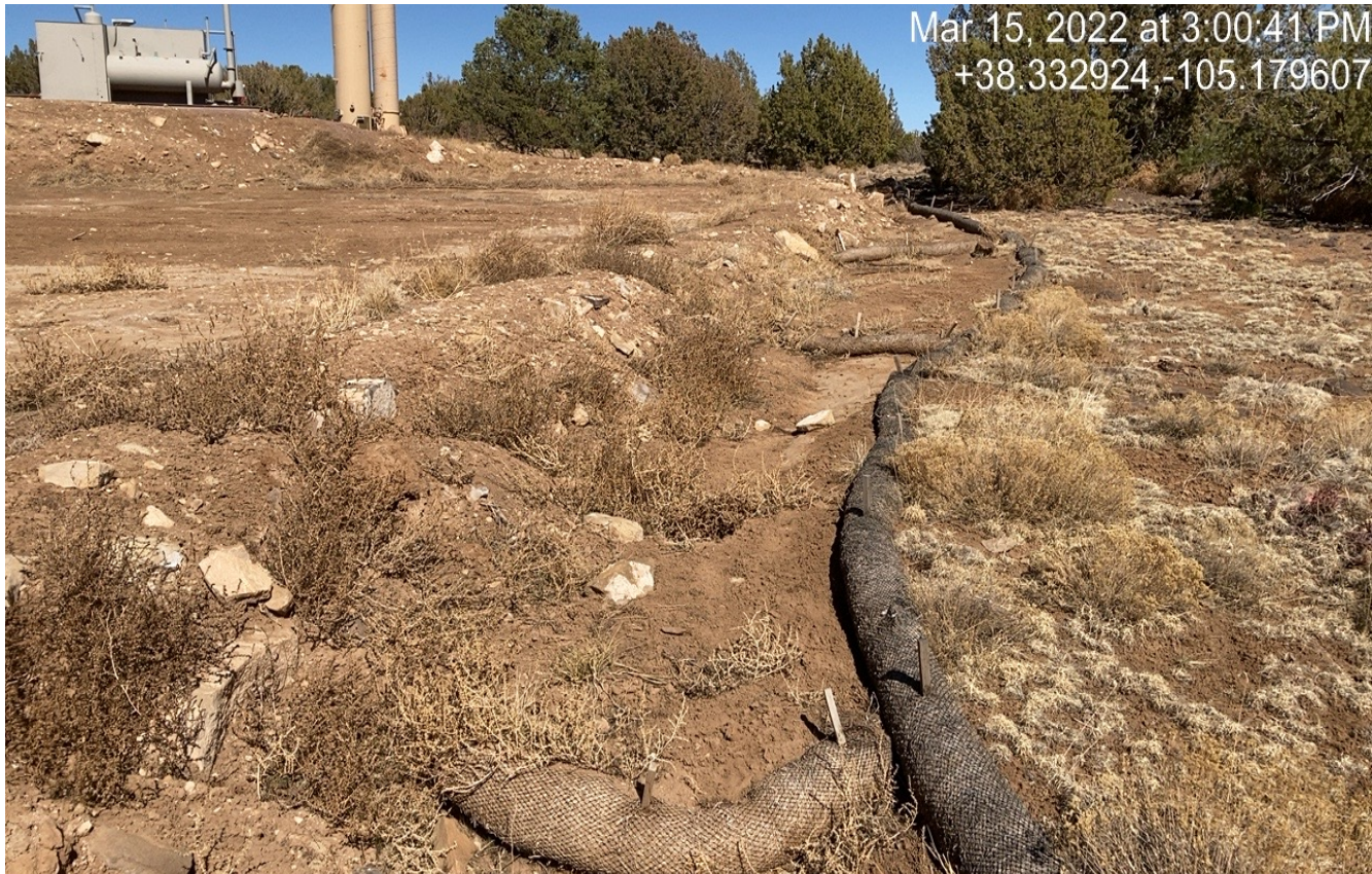
Photo 5. The wattles are degraded and are filled in with sediment. Previous corrective action has not been performed.
