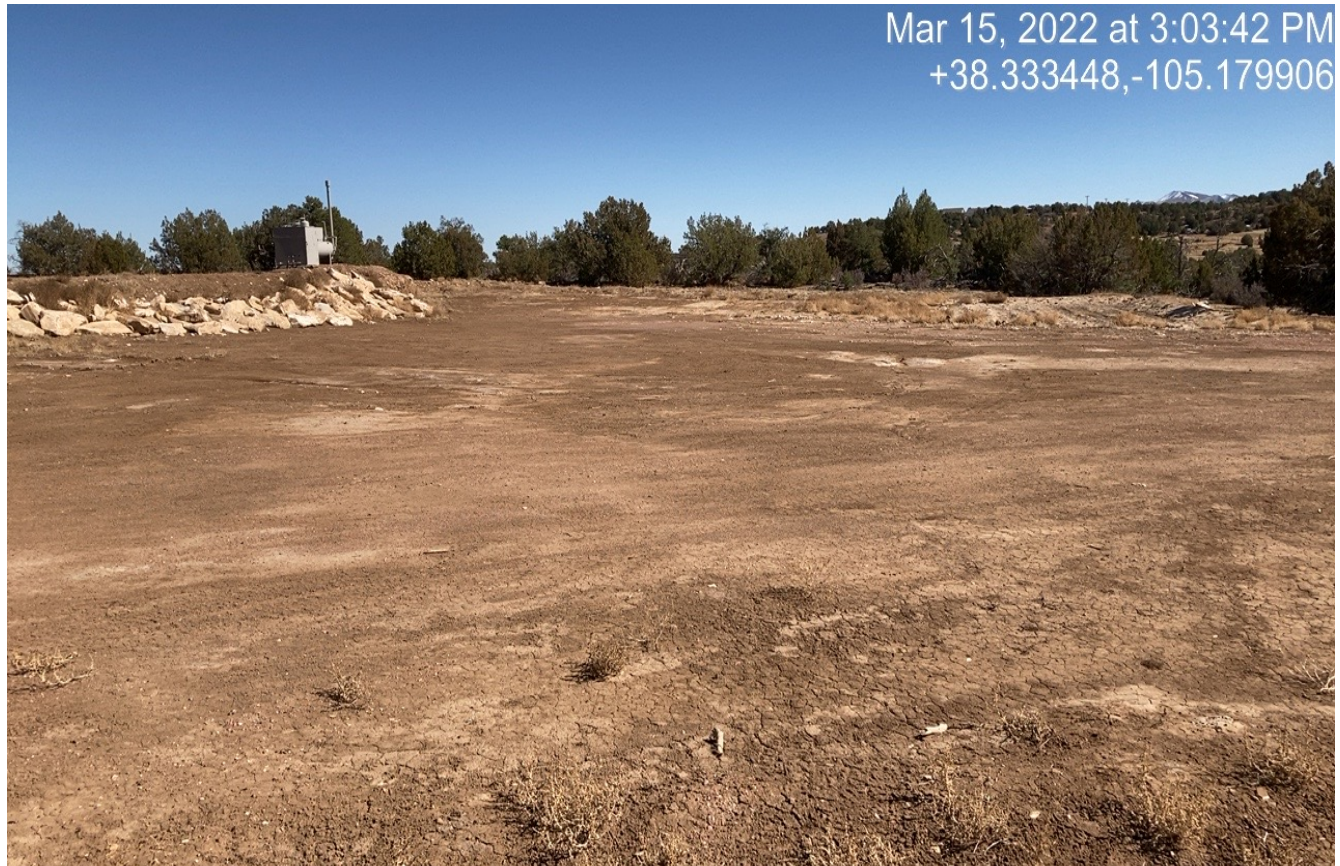
Photo 12. Facing northeast toward the location. Unused areas of the location need to be recontoured and reclaimed. Previous corrective actions have not been performed.
