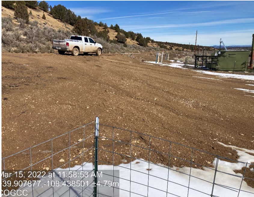
Lack of stabilization-compaction
