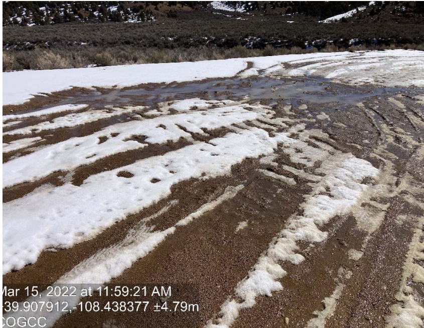
Lack of stabilization-compaction
