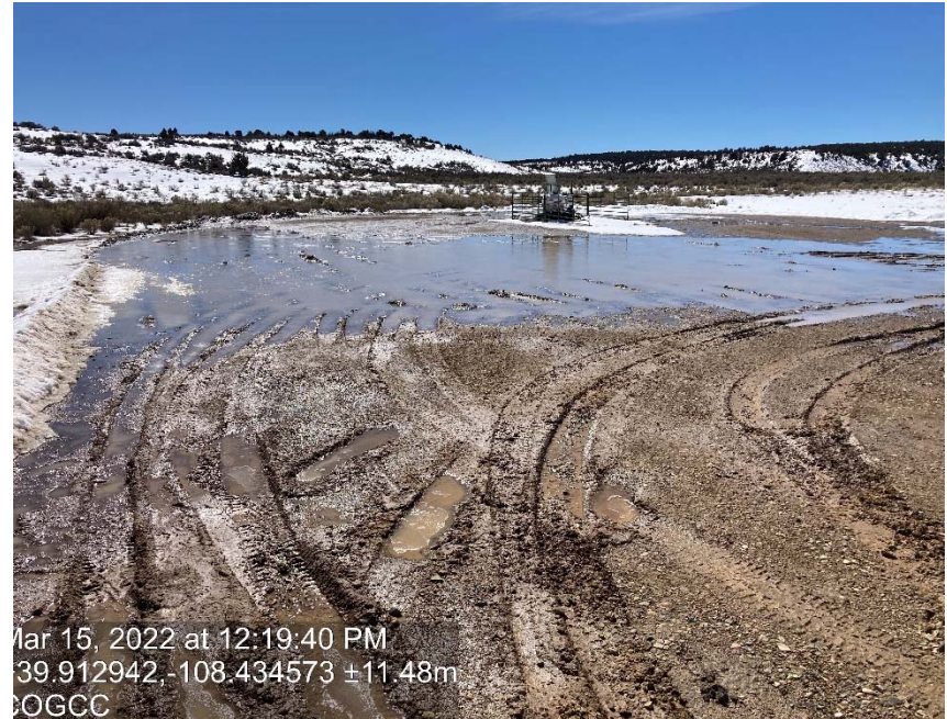
Lack of stabilization-compaction
