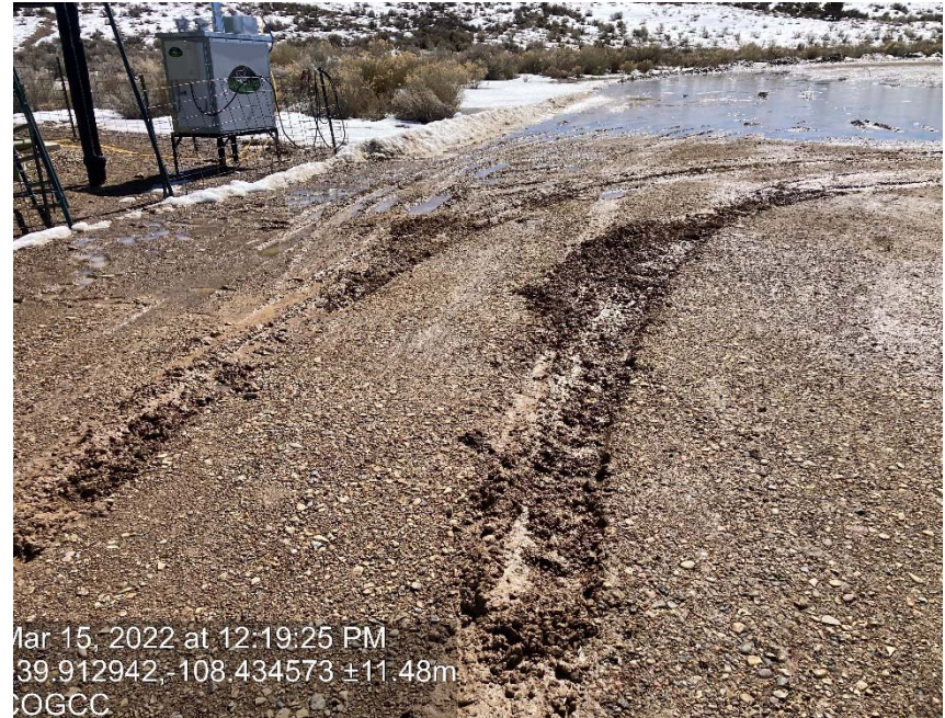
Lack of stabilization-compaction
