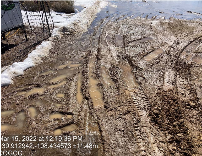
Lack of stabilization-compaction
