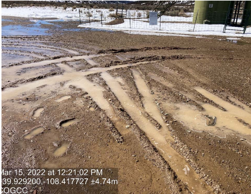
Lack of stabilization-compaction
