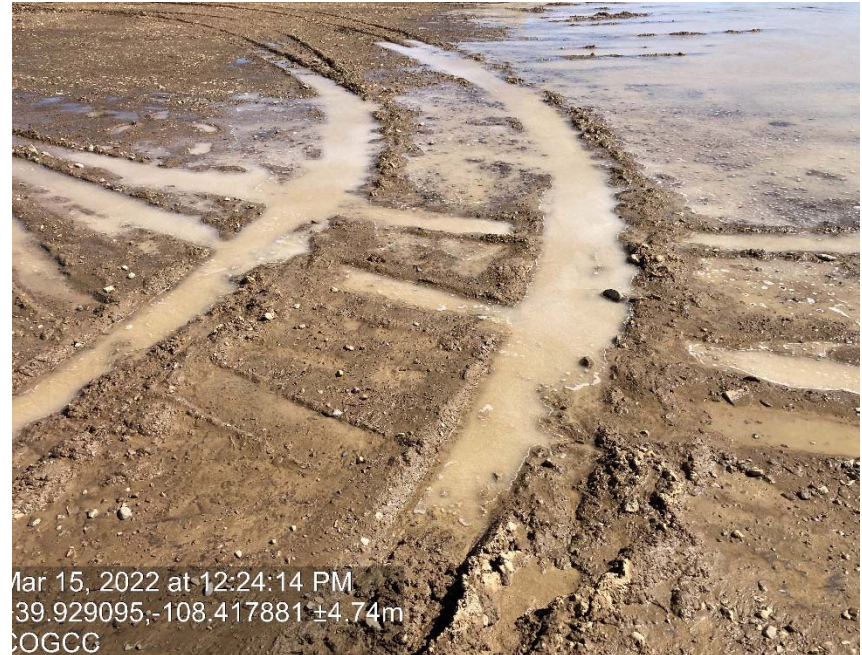
Lack of stabilization-compaction
