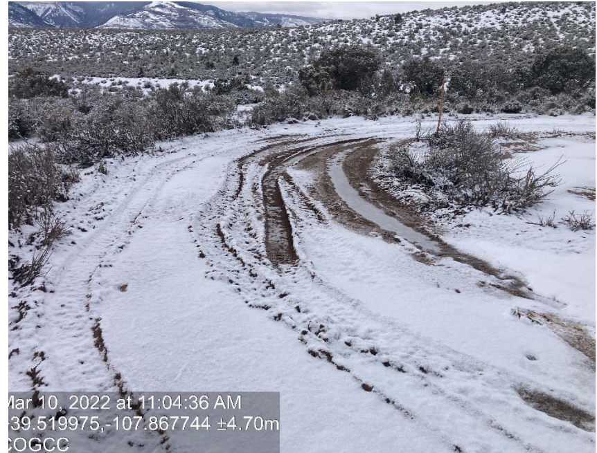
Lack of stabilization/ compaction
