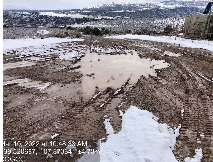
Lack of stabilization/compaction
