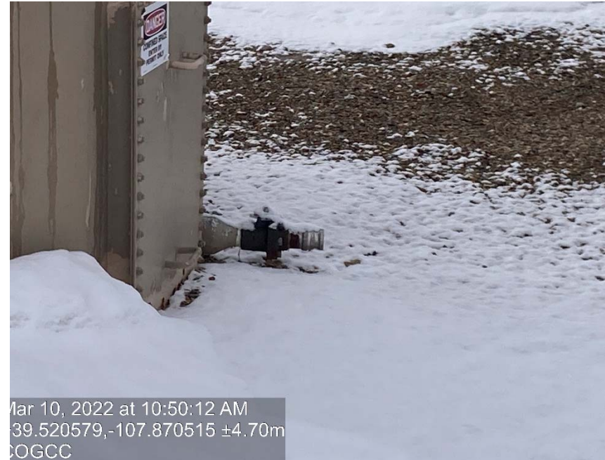
Lack of cap (Cam lock)
