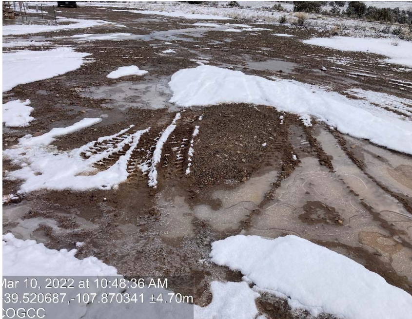
Lack of stabilization/compaction
