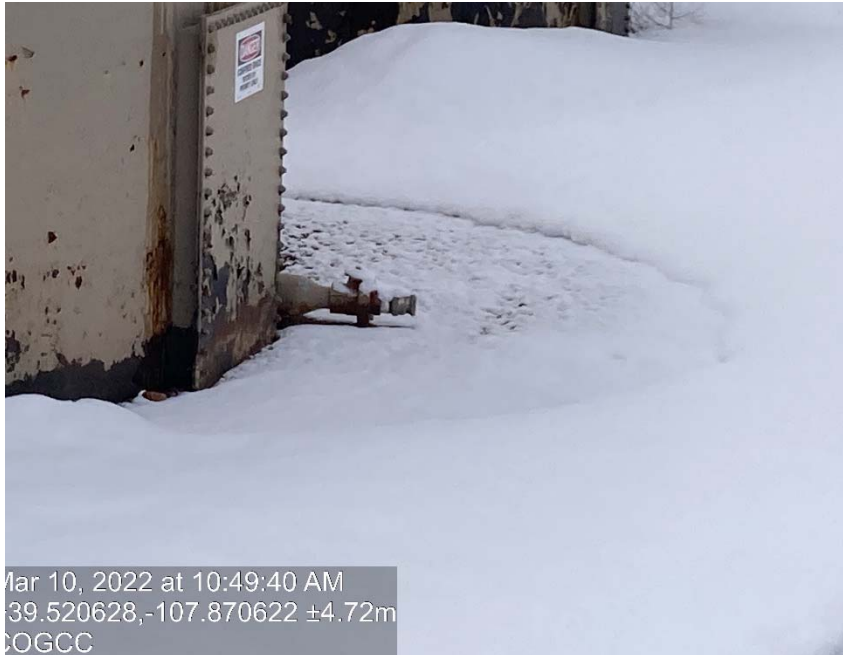
Lack of cap (Cam lock)
