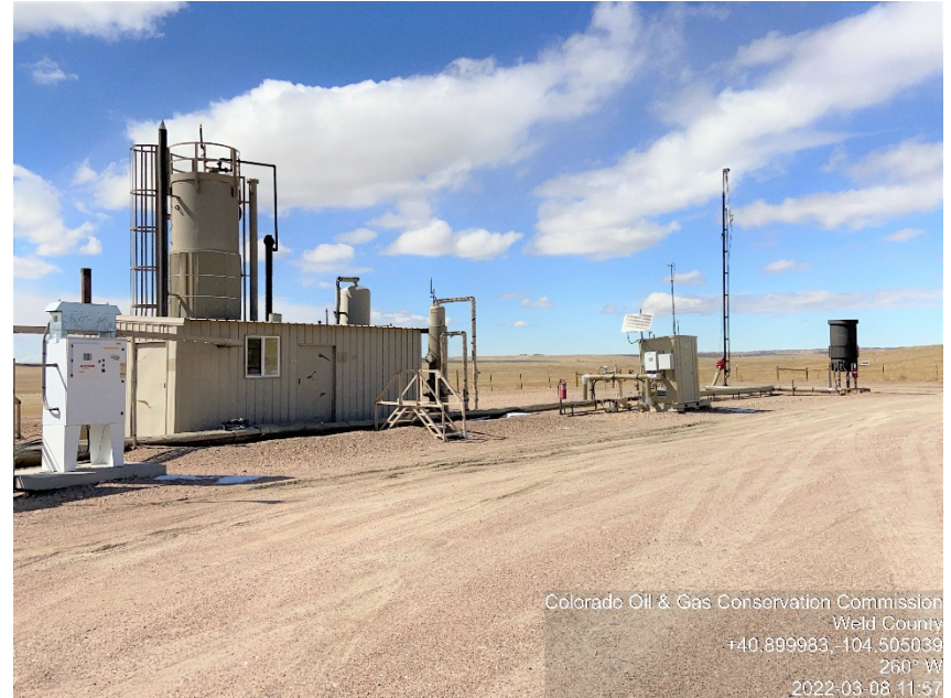
Photo #4 Lion Creek 02-13 Battery site Active Treater, Separator, ECD
