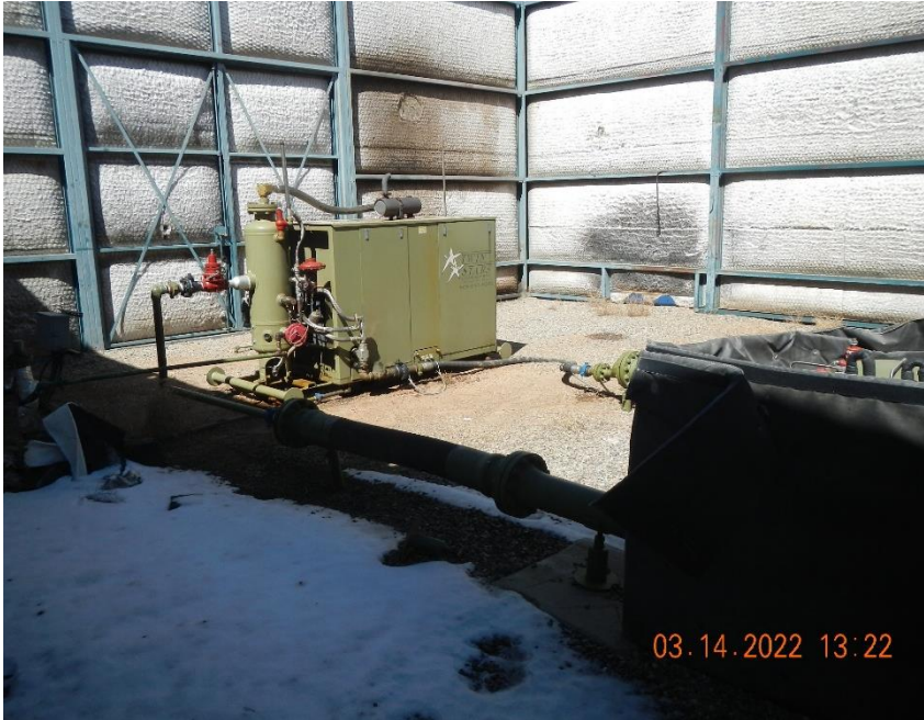
Compressor within sound walls.
