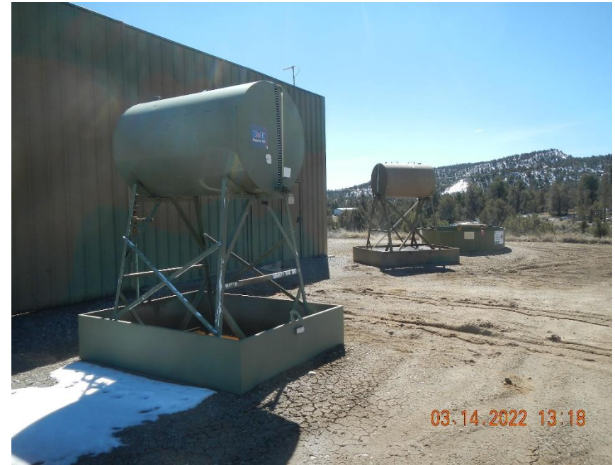
Lube oil containers and produced water PBV with secondary containment.
