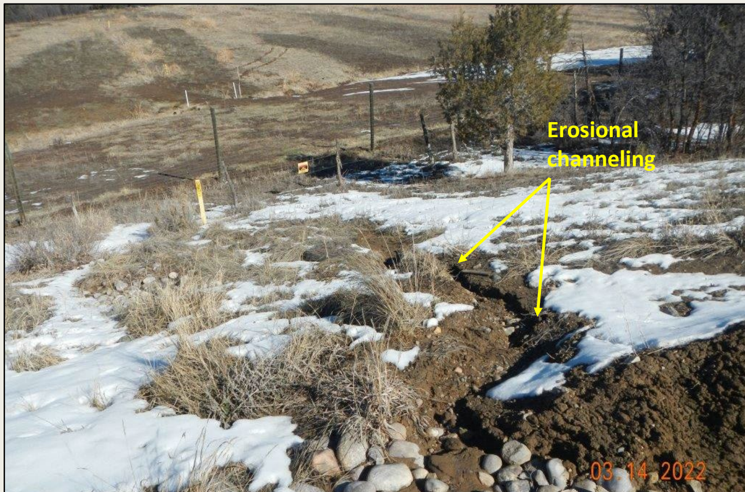
Photo 4. View of area in the northern project area where stormwater flows around a cobble BMP and is eroding the fill slope.
