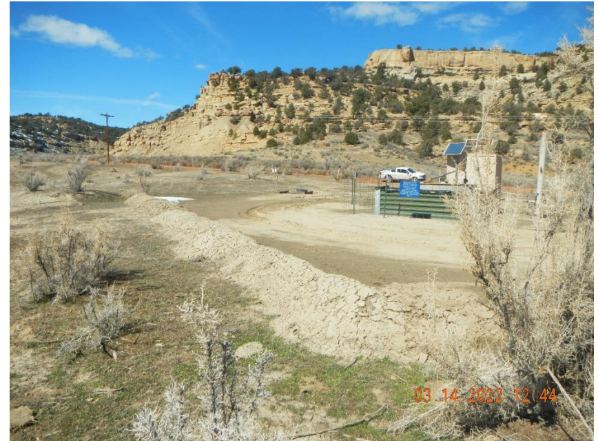
Berming installed to prevent run off erosion.
