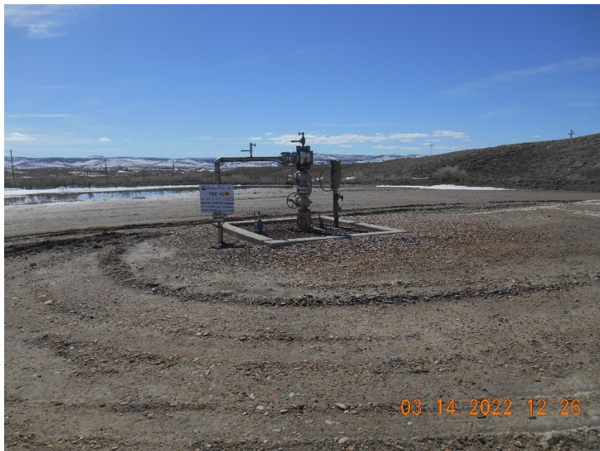
Injection wellhead
