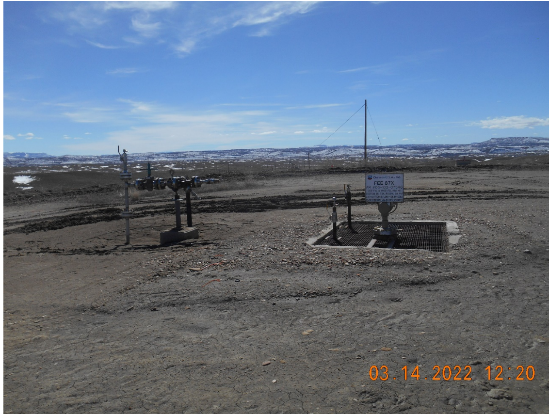
Injection Wellhead – Temporarily Abandoned
