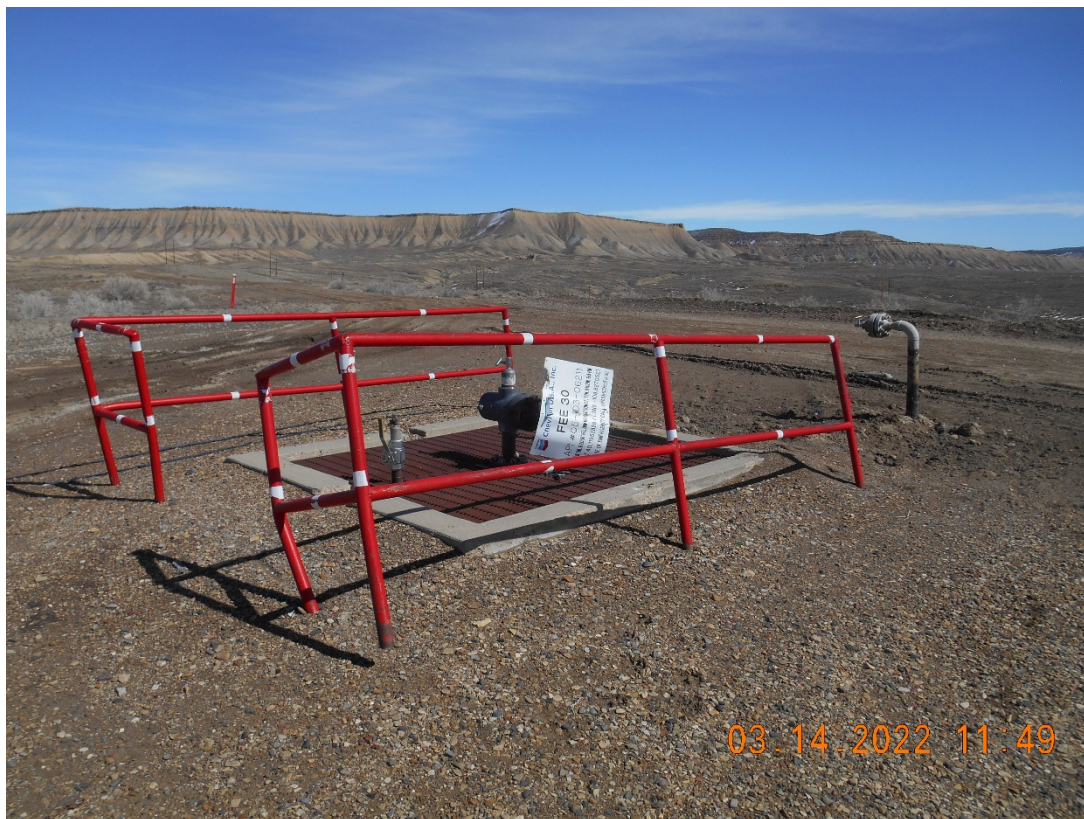
Injection wellhead – Temporarily Abandoned
