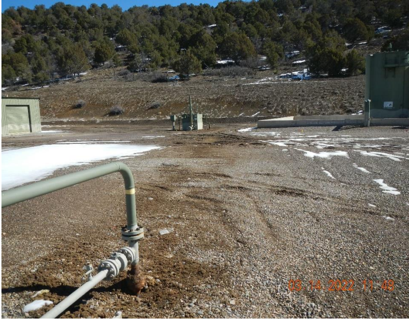
Spill/Release Point ID #480565 point source. Flow line excavation path visible between well head and separator.
